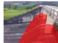
Heightening of Spillway of Sul Dam (Heightening by 2.0 m)
