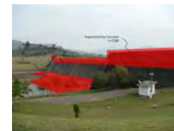
Heightening of Oeste Dam (Heightening by 2.0 m)
