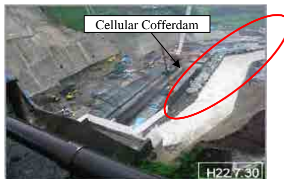
Figure 7.2.4 Example of Construction Cellular Cofferdam
