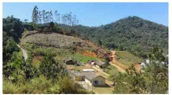
The slide of the yellow-reddish soil distribution area of the southwest region of Pomerode was activated at the end of August 2010 and has destroyed 2 houses near the hillside. The surrounding area of the two residences was a swamp until 25 years ago, and soft ground. The slide activated in the drought season. The slip surface is in red-yellow acrisols soil had been deteriorated over the years, and activated by slip surface to be below share strength.
