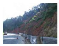
Source: JICA Survey Team, May 26, 2010 Site of a disaster prevention work in the municipal road of Blumenau, executed by DEINFRA. Collapse of the thin layer of yellow-reddish soil that covers the base rock.
