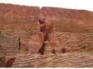
Source: JICA Survey Team, May 08, 2010 Erosion in the yellow-reddish soil on cut slope in the municipality of Pomerode. It easily becomes deteriorate with the infiltration of water, becoming erosible.
