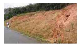
Road section between Luis Alves - Massaranduba of the state road SC413 in the municipality of Luis Alves. There is a sliding face within the yellow-reddish soil. In the rainstorm of November 2008, it completely obstructed the road. The sliding face is located a little above the road surface, and even now, a stretch 60m long along the road is advancing to the road. The total length, including the non-activated part, is 240m.
