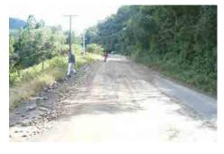
Slide of the pelitic sedimentary rock distribution area of the Mesozoic era on the state road SC302, upstream the dam of Itajai do Oeste river, in the municipality of Taio. The road corresponds to the slide head, and at the left side of the photo there is the river, and in the hill at the right side we can observe the distribution of phyllite with water spring.
