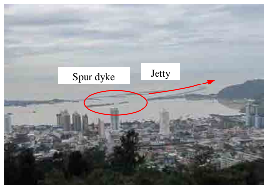
Jetty and Spur dyke in River Mouth
