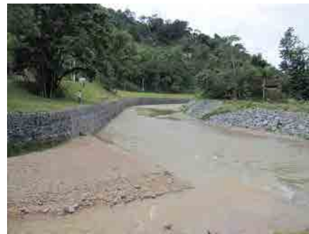
Gabion works after the 2008 flood damage in the Garcia River, Blumenau city
