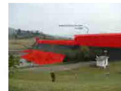
Heightening of Oeste Dam (Heightening by 2.0 m)
