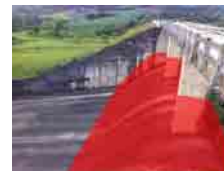
Heightening of Spillway of Sul Dam (Heightening by 2.0 m)
