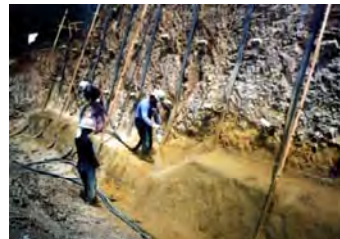
Example: Soil Splaying with PP fiber/cement/sand mixture under construction
