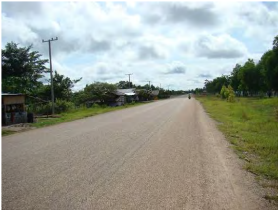
Around Xeno Route passing the lowland and flat land. Almost no cut slope or embankment, with gentle alignment
