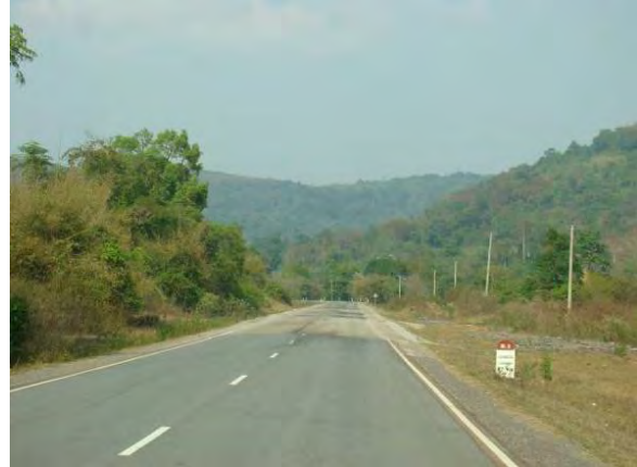
Around Den Savan Route passing through mountainous areas. Road with many cut slopes. Alignment including many curves along the land features
