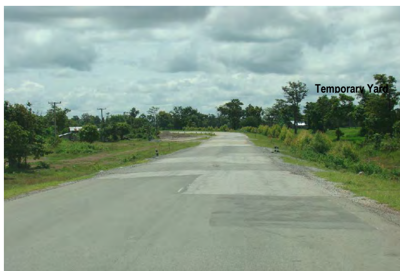
Figure 2.2.23 Condition of the temporary yard candidate site (at around KM70 point)
