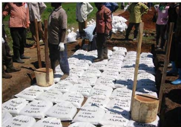
Figure 8-20: Sandbag Technology of Road Rehabilitation (Image)
