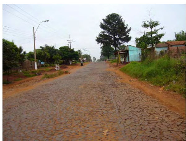
Typical Stone Pavement Section near the Ciudad del Este (Parana River Coastal Road)
