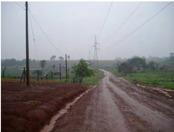
When it rains, road condition become worse and it will be hard to traffic (Parana River Coastal Road)
