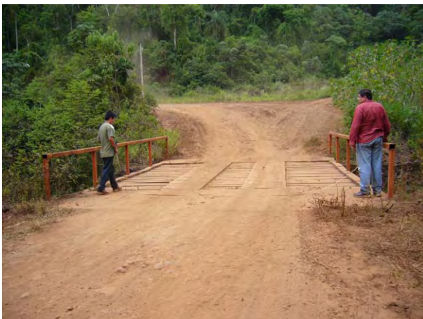
Bridge on the Port Access Road (to Pt. Torocua)
