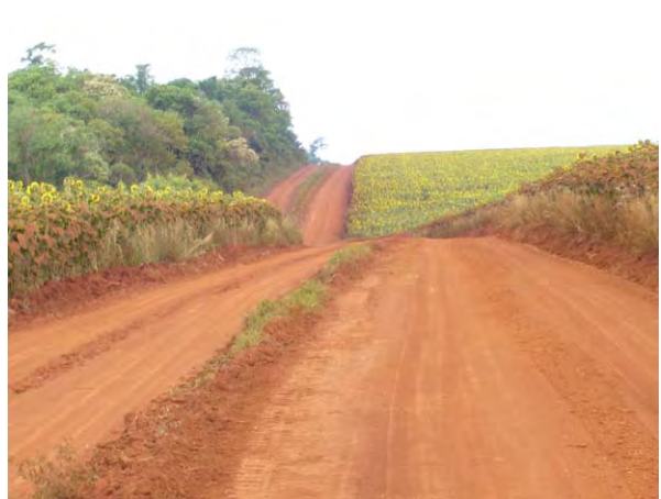
Rolling Port Access Road (to Pt. Paloma)
