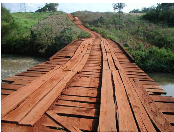
Timber Bridge crossing the Yacuy Guazu River (Parana River Coastal Road)
