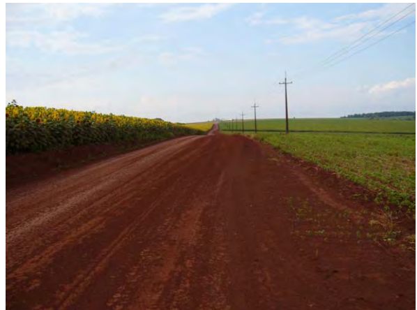
Typical cross-section of the National Road Route 6 - Coastal Road Connection Road (Dirt Section)
