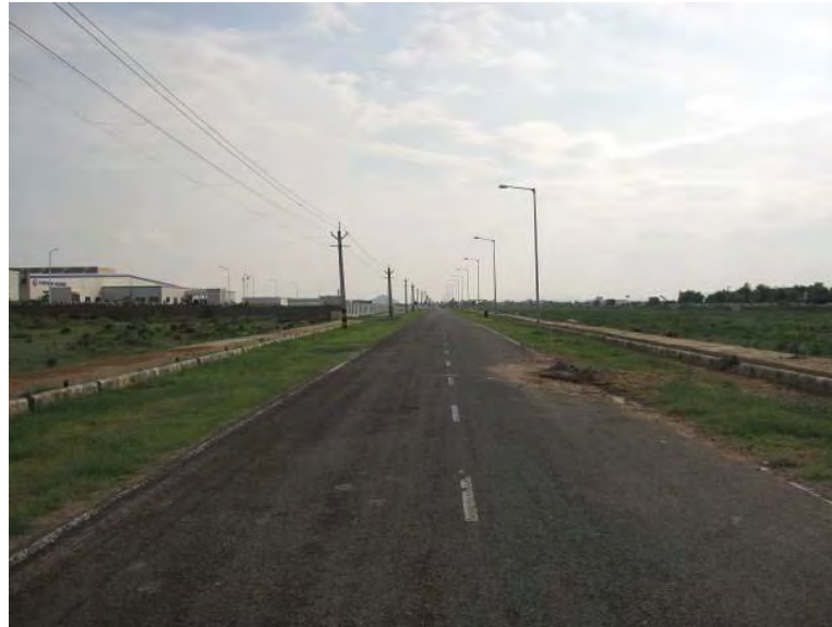
Fig. 7.4-1 Road Condition in the NIC
