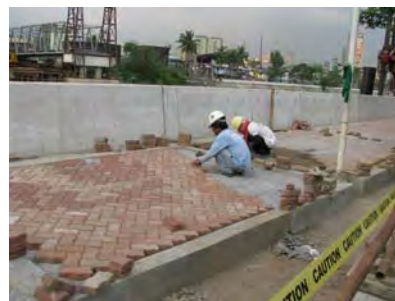
(Completed Revetment and River Wall)
