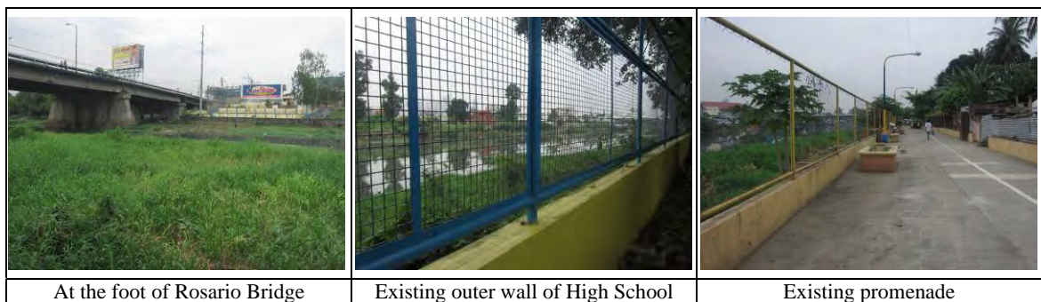
Figure 5 Existing Condition of Lower Marikina River
