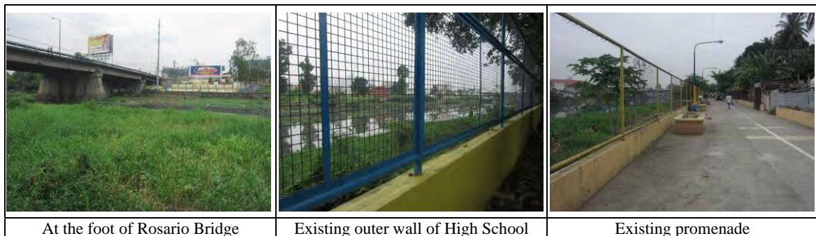
Figure 3.5.5 Existing Condition on Lower Marikina River
