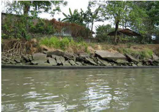
Damaged Bank Protection Works (Pasig River)
