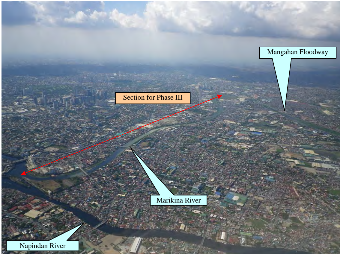
Phase III of Pasig-Marikina River Channel Improvement Project (Photo taken in 2009)
