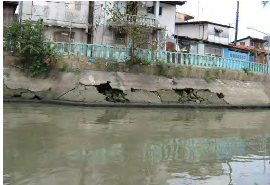
Damaged Bank Protection Works (Pasig River)
