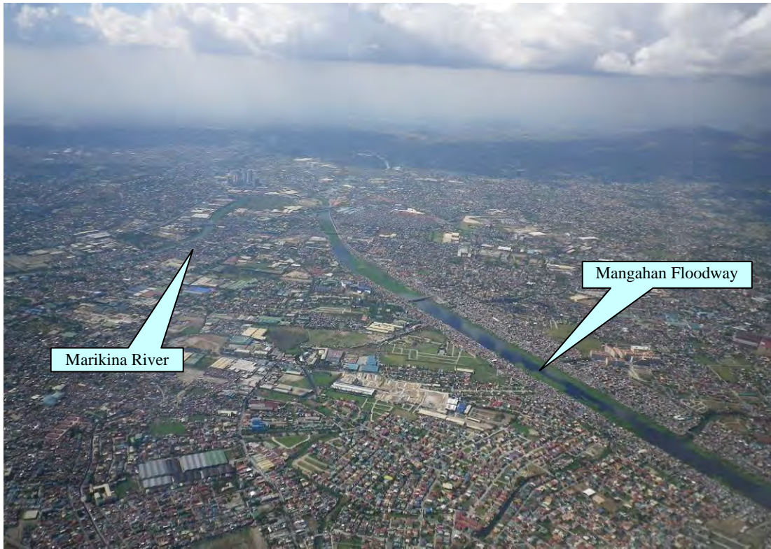
Mangahan Floodway and Congested Residential Area (2009)
