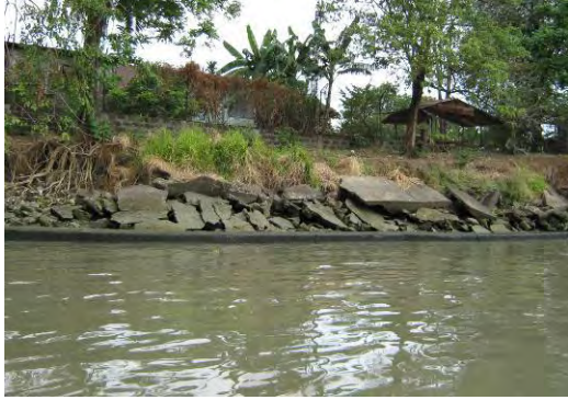
Bank Protection Works Damaged after D/D (Phase-II Area)
