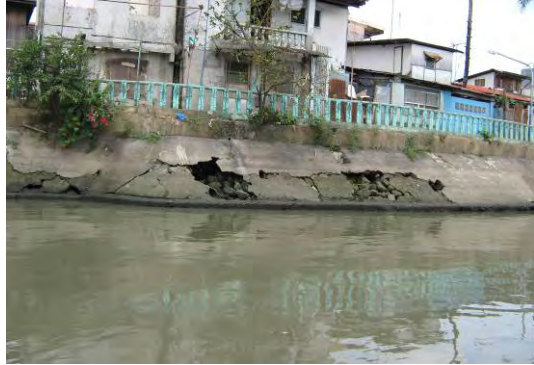
Bank Protection Works Damaged after D/D (Phase-II Area)
