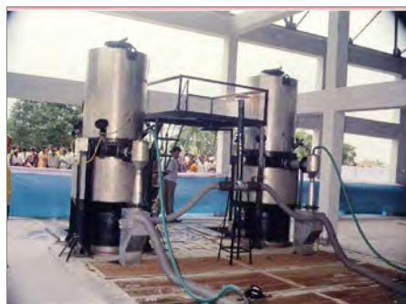
Figure 4.4 Biomass Gasifier Plant
