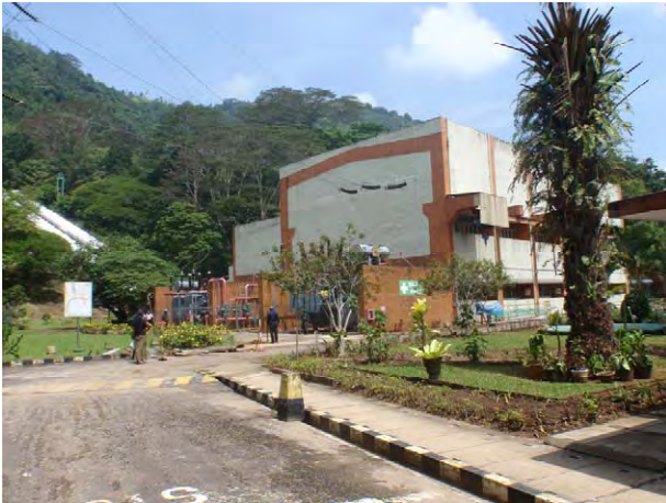
Ukuwela HPP (2 × 19 MVA)
