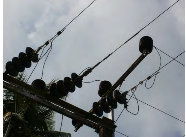
Connection of 33 kV Distribution Lines
