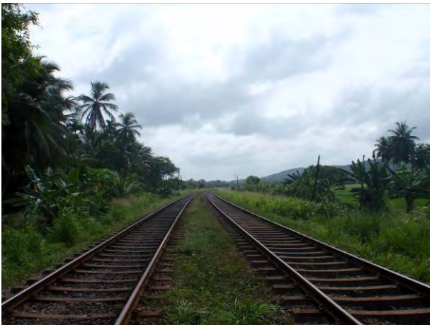
Railway Crossing Point in Route of New 220 kV Habarana-Veyangoda Transmission Line
