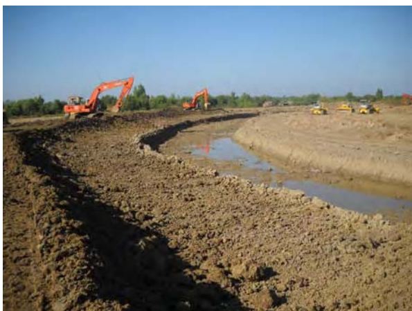
Polder Dike Rehabilitation Work Under machine embankment work.
