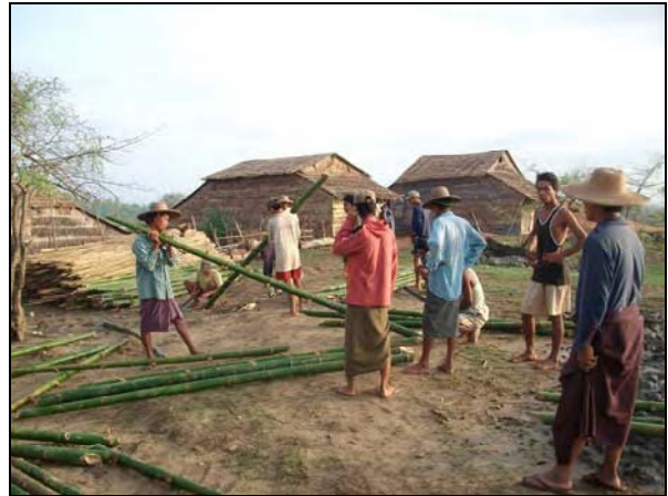
Mangrove Windbreak Project Preparation of tide protection fence using bamboo by villagers (May 2010).
