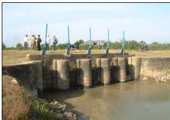
Present Condition of Existing Sluice: Slide Gate Side (January 2010)
