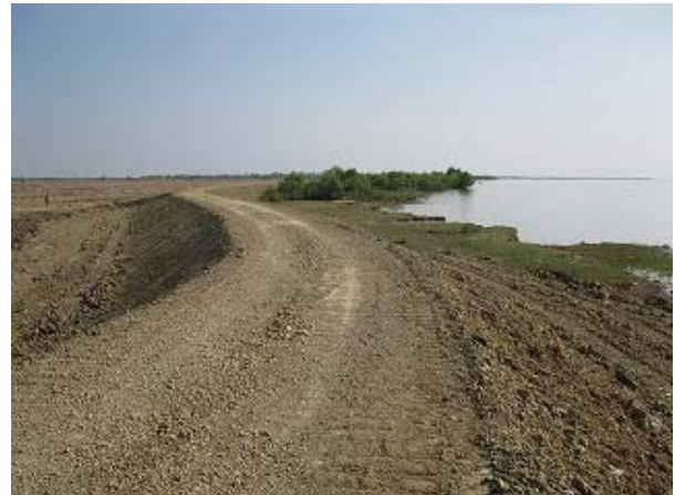
Polder Dike Rehabilitation Work Completed by ID in March 2011.
