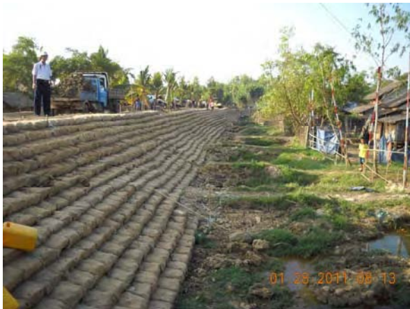
Polder Dike Rehabilitation Work Manpower Embankment near houses (January 2011).
