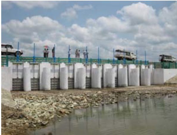
Sluice Rehabilitation Work Completion inspection at Hpobe Sluice (31 March 2011).
