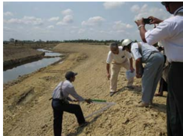
Polder Dike Rehabilitation Work Completion inspection (31 March 2011).
