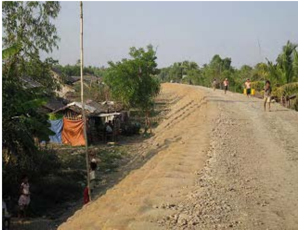
Polder Dike Rehabilitation Work Completed with manpower embankment.
