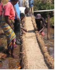
If stone is not available in and around the site, even banana sheath can be used as a temporal material for ditch lining in order to prevent soils from being eroded.
