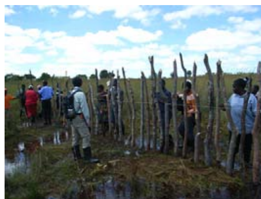
Using a string to align the poles
