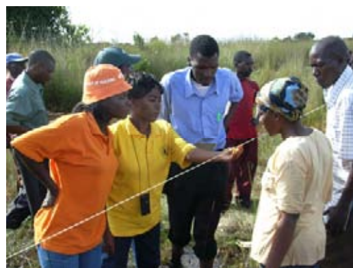
Deciding an canal alignment with a line level
