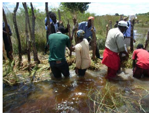
Compacting the basement of the weir
