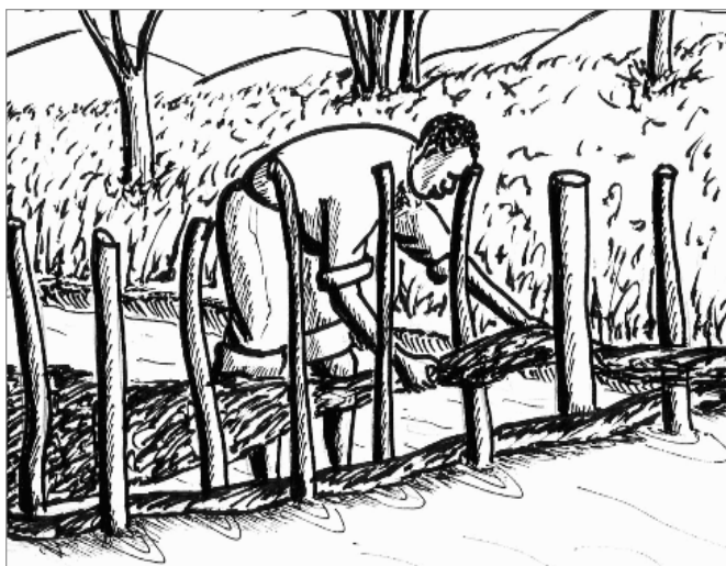
Single-line diversion weir
