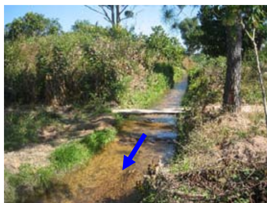
Community based or individual small-scale irrigation schemes were established since 1940s in the earliest. In most cases, locally available material are used for making of river diversion weir as a temporarily facility. Right: Temporal weir, Left: furrow led to irrigated area. (May 2009, Mungwi District)
