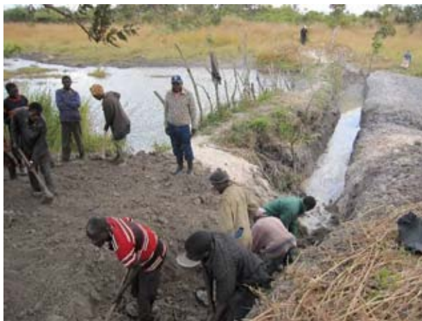
The participants are digging core-trench of the small earth dam. (As of mid-July 2010).
