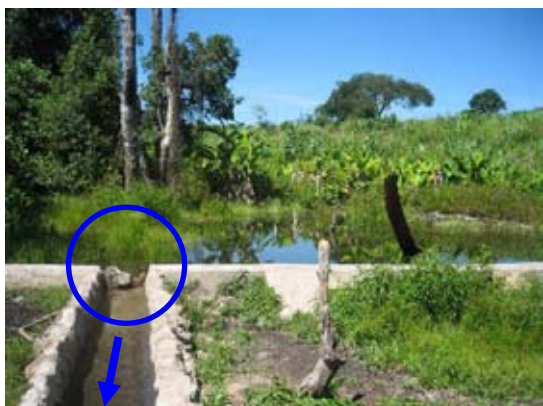
A permanent weir without any water control devices like a gate. The users put stones at the outlet of the weir as to operate amount of water flowing into the furrow. (June 2009, Mungwi District)
