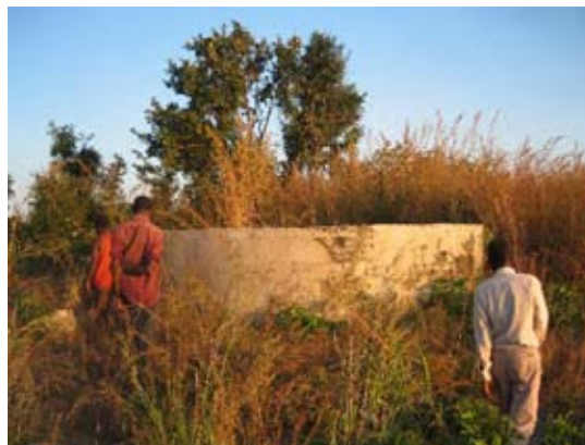
A pump irrigation site suspended its operation in 2002 due to deficit of water volume to be lifted up and lack of knowledge to repair pump equipment. Left: Engine pump provided in 1997, Right: Water tank not utilized any longer (June 2009, Kasama District)
