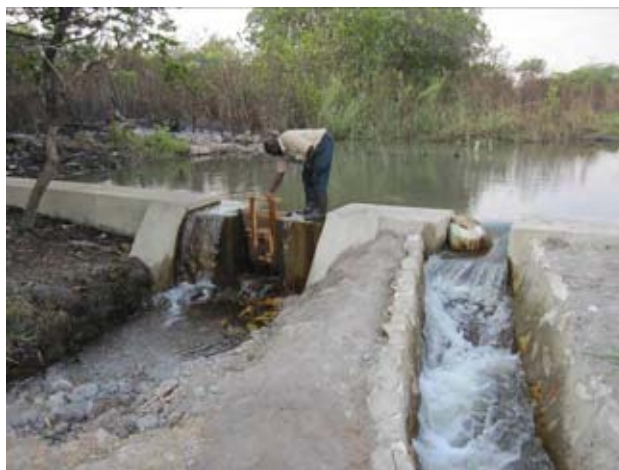
The weir equips a sand sluice gate (Center) from environmental aspect, which is expected to work to flush the sand accumulated in the water pond and to let a small fish go upstream. (As of late in September 2010)
