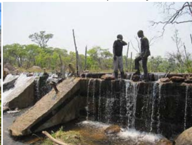
In year 2010, by improving the remaining temporal parts, all the parts of the weir has at last been graded up from temporal to permanent. (As of late in September, 2010 )
