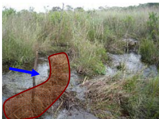
Community based or individual small-scale irrigation schemes were established since 1940s in the earliest. In most cases, locally available material are used for making of river diversion weir as a temporarily facility. Right: Temporal weir, Left: furrow led to irrigated area. (May 2009, Mungwi District)
