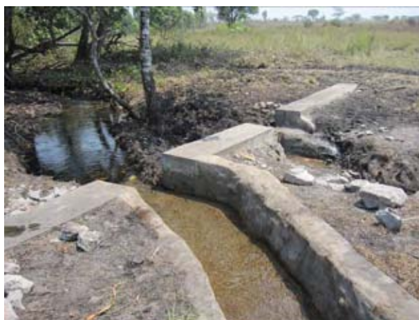
The masonry type weir constructed by Chaiteka community people under the supervision of Luwingu TSB staff. The members now enjoy irrigation farming with the water diverted by the new permanent structure. (As of the end of September in 2010).
