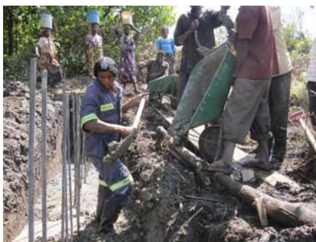
The construction stage is to place concrete for foundation of the weir (Nseluka site, as of mid July).
