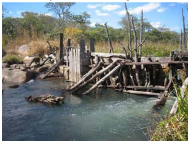
Since 2006, year by year, the farmers of the site have continuously reinforced the temporal weir by using foreign materials like cement and iron bars which have been contributed by members themselves. (As of July 2009).
