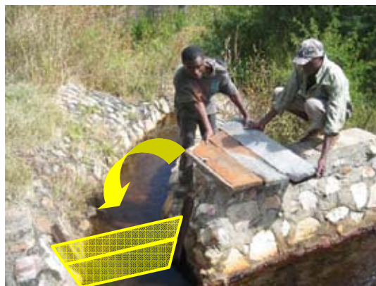
A permanent weir equipped with stop-log gate of timber board. The farmers operate the gate to adjust water volume for meeting water requirement on the irrigated field, (June 2009, Chinsali District)
