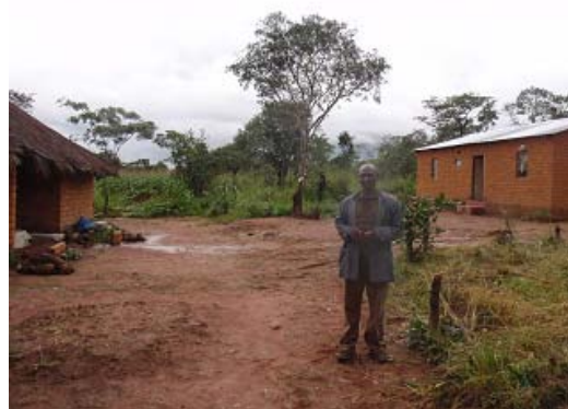
Famer stands in between old thatched house (left) and newly constructed house with iron sheets after COBSI introduction.
