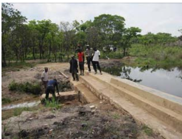
The masonry main body has completed. The persons concerned such as the community members, TSB staff, and skilled labors are finally checking the details of facility. (As of early in November, 2010)
