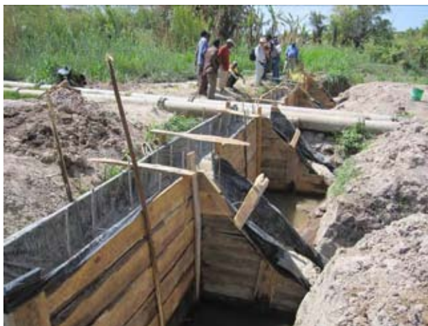
The construction reached the final stage to place concrete to last layer. After that, the construction was successfully finished and then the weir has started supplying enough water to irrigated plots being cultivated by 53 farmers.
