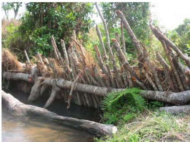
An example of an inclined weir: a large log is laid across the river and, to raise the water level, branches, grasses, and clay soil are placed in front of it, which is further supported by supporting logs from behind.
