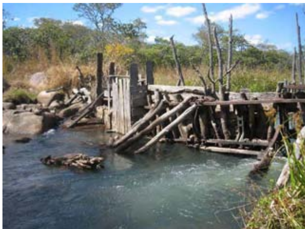
Since 2006, year by year, the farmers of the site have continuously reinforced the temporal weir by using foreign materials like cement and iron bars which have been contributed by members themselves. (As of July 2009).
