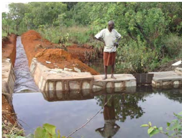
A masonry type of weir constructed under 2010 pilot project has started supplying the irrigated land with water (As of mid-November 2010).
