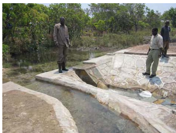
Wet-masonry-type permanent weir, upgraded in 2010 from a temporary one: originally, only the right bank of the stream was being irrigated, but through upgrading, intakes were installed at both sides so that farmers on the left bank can also enjoy the irrigation.
