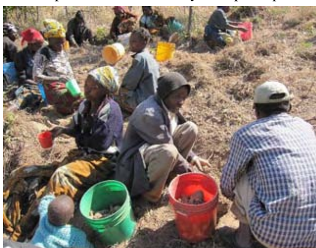
The scheme members are collecting stones for making concrete as preparation work to next stage. (Malashi site, as of the end of June, 2010)
