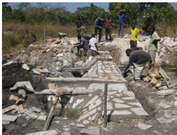
The masonry type of weir has been almost piled up on the Kasakalabwe stream, Mporokoso district (as of mid July)
