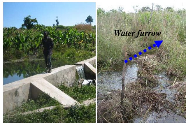
There are mainly two types of irrigation scheme: left photo is a typical concrete weir, a permanent structure, while right one is a temporary stoppage
