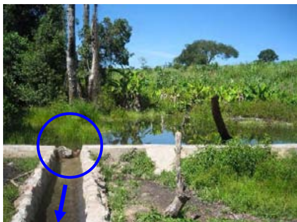
A permanent weir without any water control devices at the intake. The farmers usually put stones at the intake so as to control the amount of water flowing into the furrow. (June 2009, Mungwi District)
