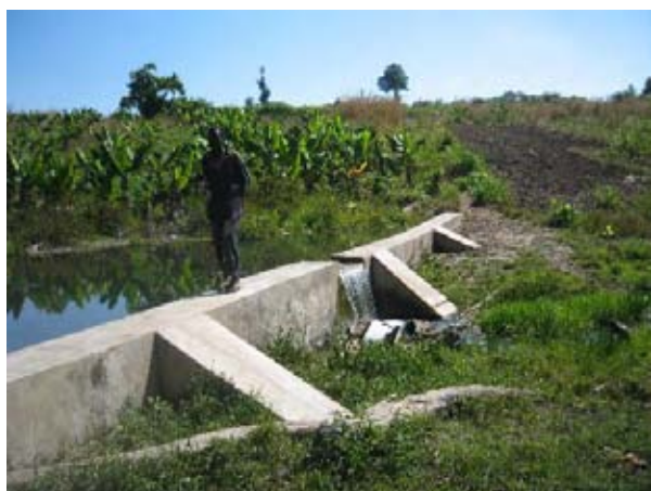
There are mainly two types of permanent diversion structures, e.g. concrete wall-type structure (left), and masonry type-wall structure (right). The former is the majority. In fact, the government started constructing such irrigation schemes in 2000s supported by donors or otherwise by utilizing the government fund.
