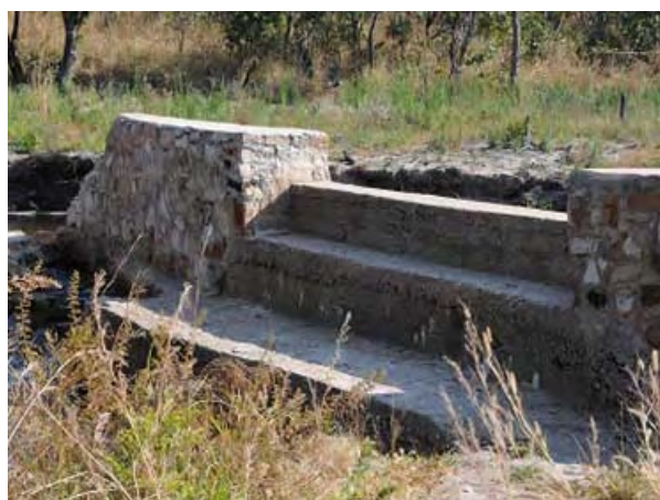
There are mainly two types of permanent diversion structures, e.g. concrete wall-type structure (left), and masonry type-wall structure (right). The former is the majority. In fact, the government started constructing such irrigation schemes in 2000s supported by donors or otherwise by utilizing the government fund.
