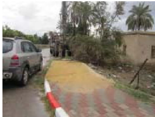
Drilling at borehole No.6 (Trunk lines)
