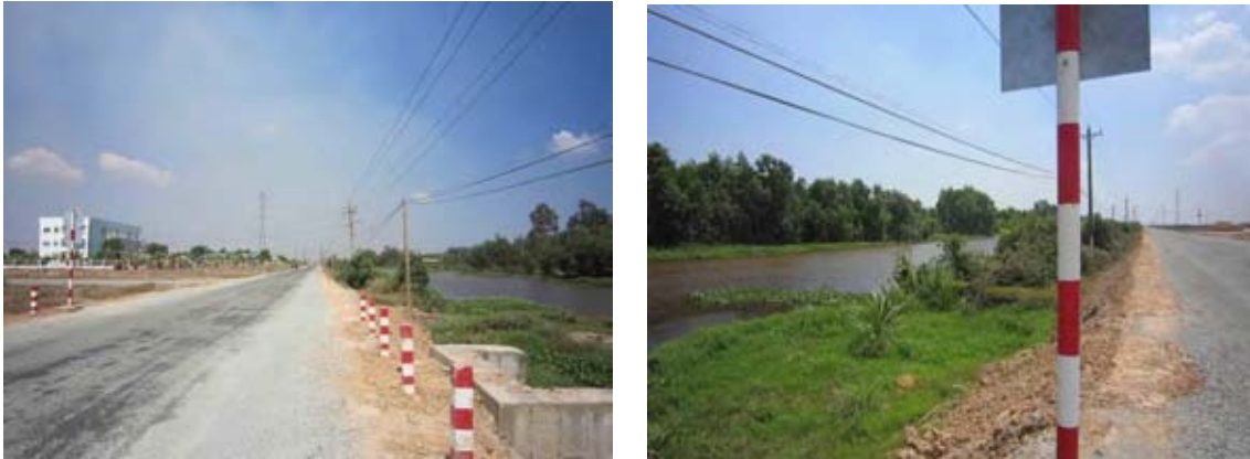
Figure 2-14 Actual state of river which is intended to use in this project in Long An province (Outward)
