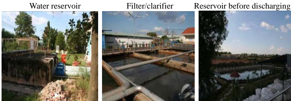
Figure 2-16 Example on wastewater treatment work in existing IP (LOTECO)
