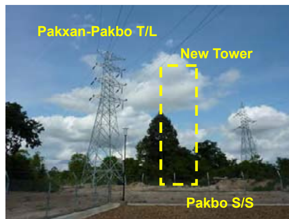
Figure 11-1 Incoming Tower Location of Pakbo Substation
