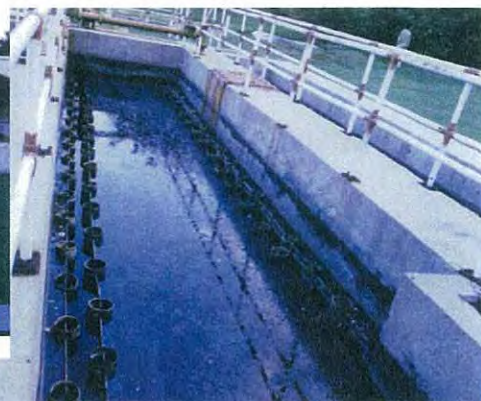
Reactor volume = 1200m 3 = 600 m 3 × 1 plus 300 m 3 × 2 Water depth: 4.5 m. HRT: 6 h. LV: 0.75 m/h
