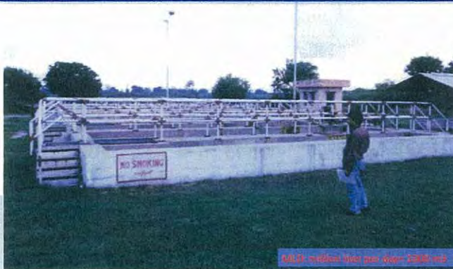
5-MLD UASB sewage treatment plant in Kanpur (1989)
