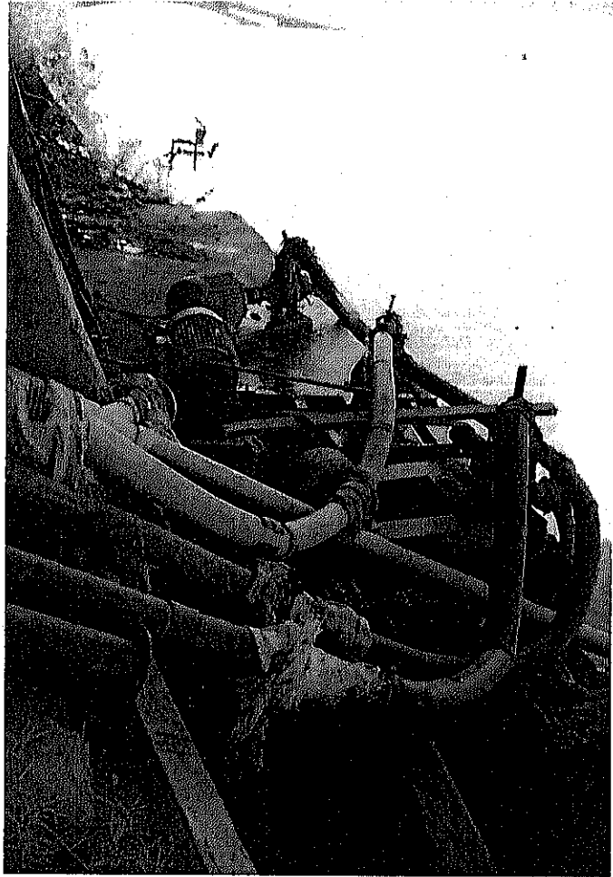
PUMP STATION NO. (2)
