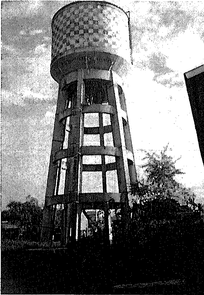
ELEVATED R.C. TANK
