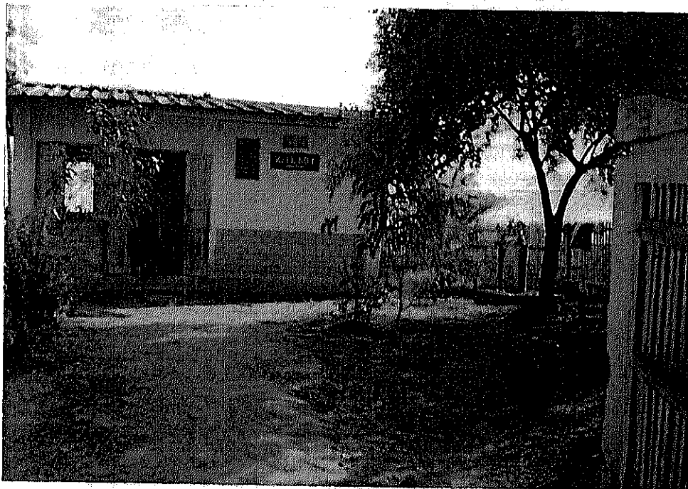
FRONT VIEW OF THE PUMP HOUSE.
