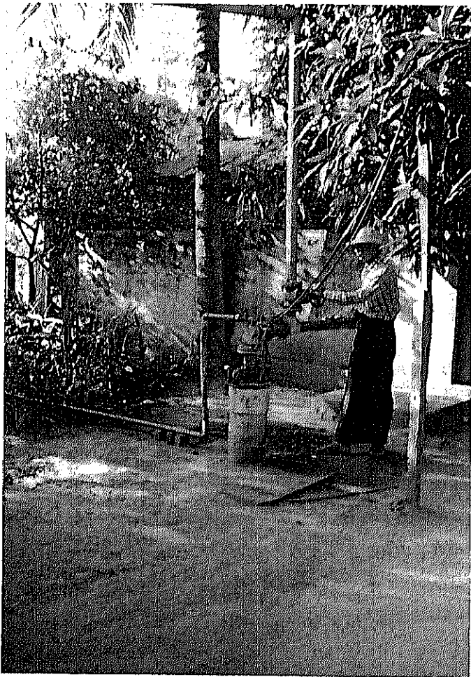
A SUBMERSIBLE PUMP INSTALLED IN ONE OF THE WELLS.
