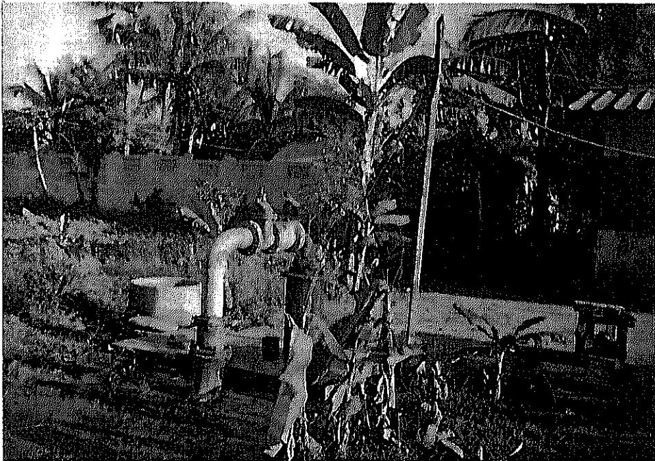
A SUBMERSIBLE PUMP INSTALLED IN ONE OF THE WELLS.
