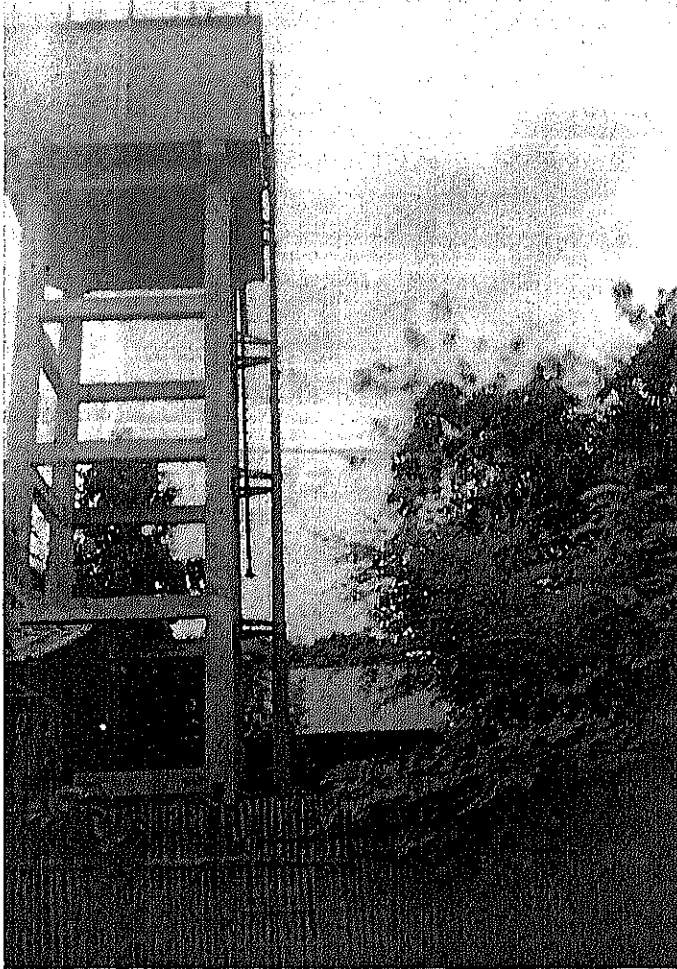
ELEVATED R.C TANK OF 12000. GALLONS CAPACITY MAINTAINED. BY THE G.A.D
