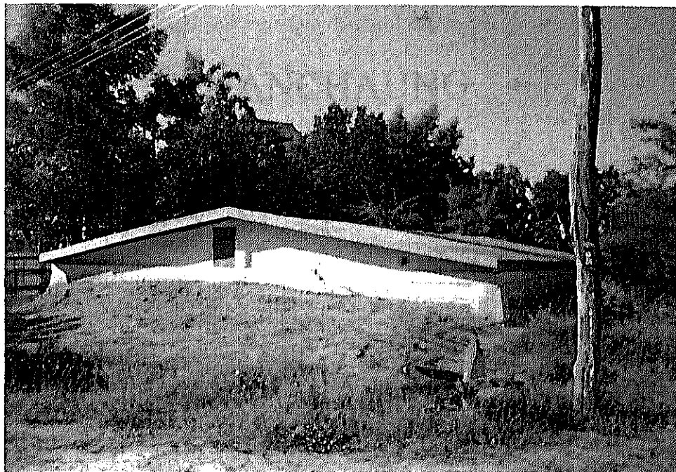
GROUND TANK OF 4000 GALLONS CAPACITY
