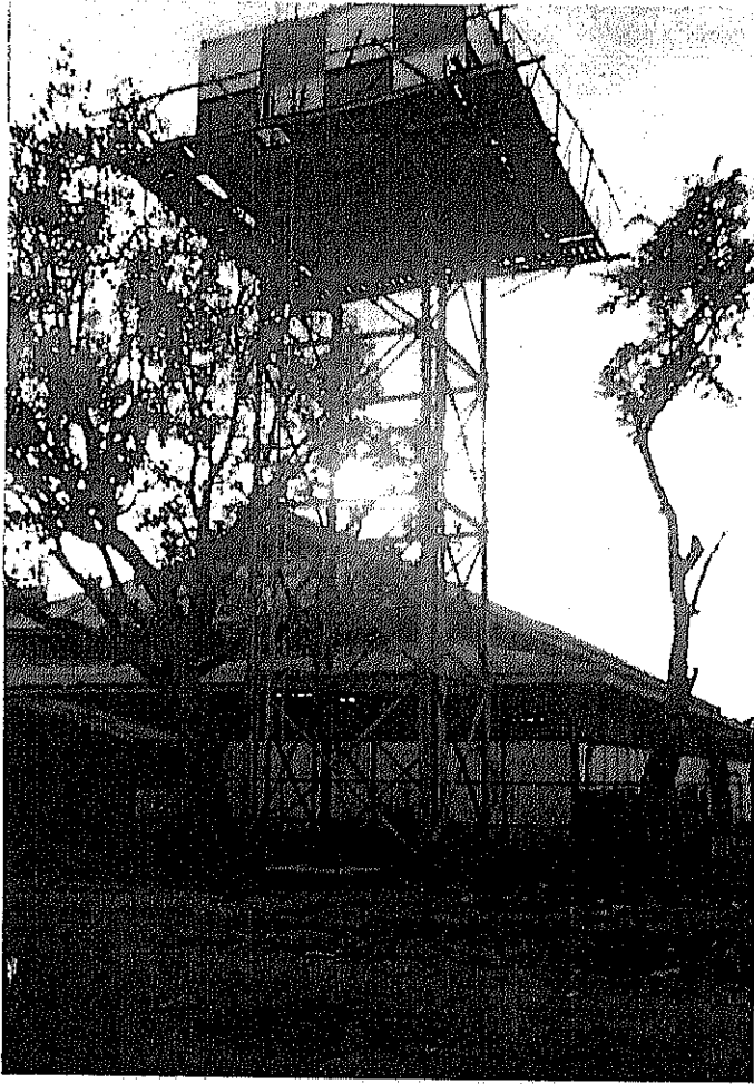
ELEVATED IRON TANK OF 12,000 GALLONS CAPACITY
