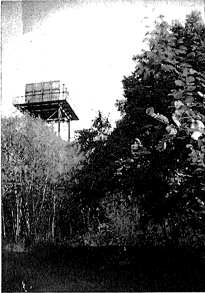
ELEVATED . F. R. P TANK 25 M 3 CAPACITY
