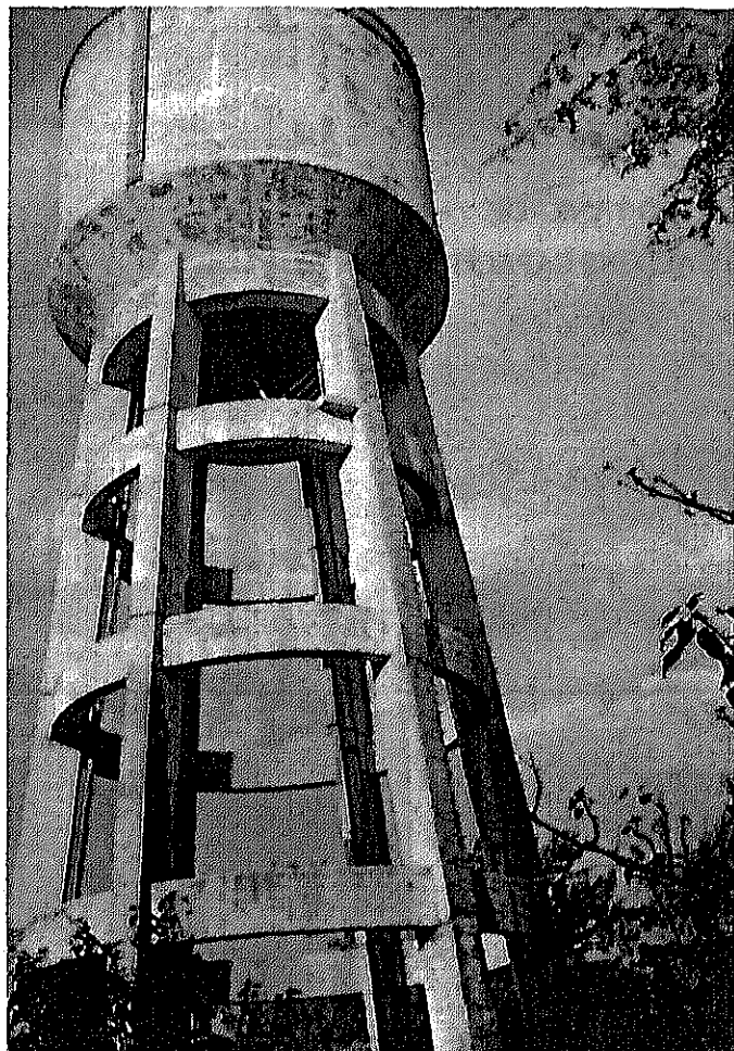
ELEVATED R . C. TANK
