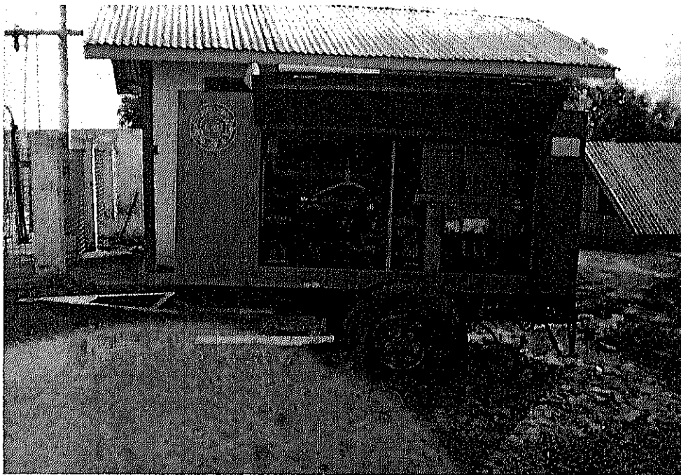
TRAILER MOUNTED, ENGINE GENERATOR 30 K.V.A. CAPACITY, OSAKA SEIMITSU MODEL "AS 3507"
