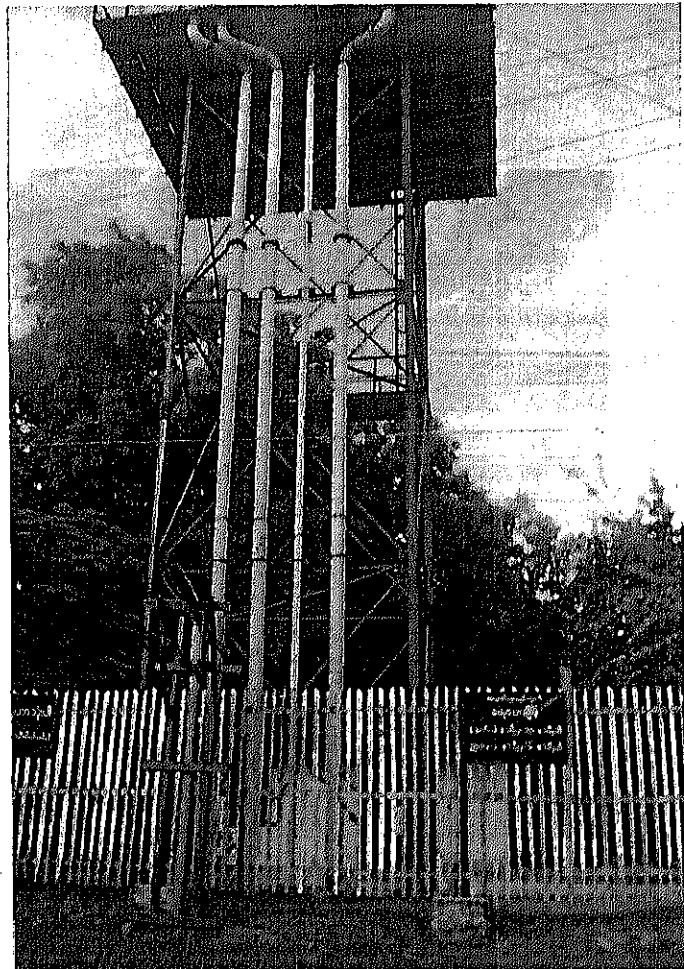
ELEVATED F.R.P TANK OF 43.3 M 3 CAPACITY.
