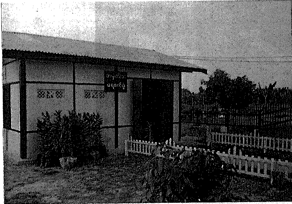
PUMP STATION NO. (1).
