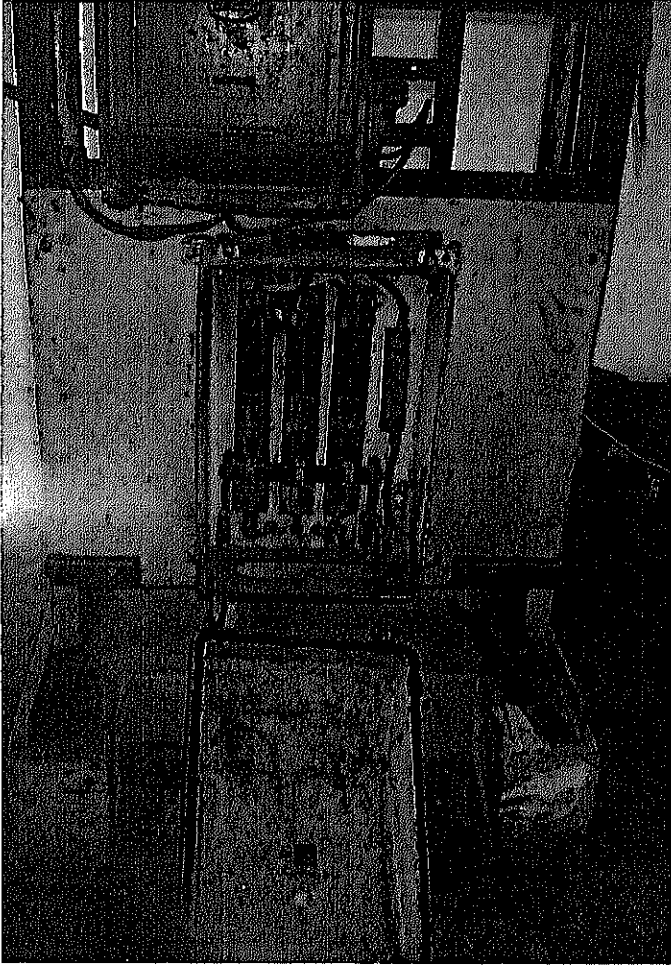
DIRECT ON LINE STARTER.
