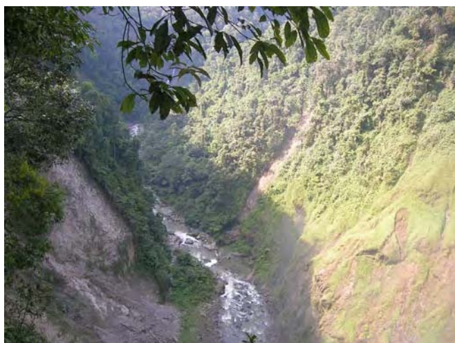
Site condition at 100m upstream from the intake area
