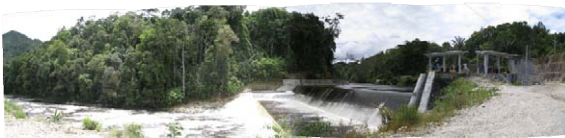
(The intake for the IPP)
