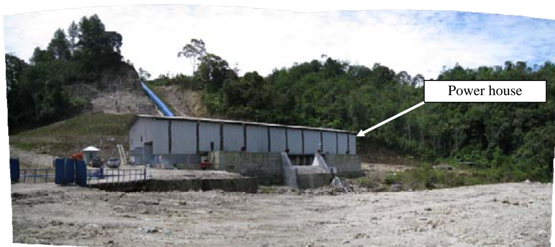
(PH under construction)
