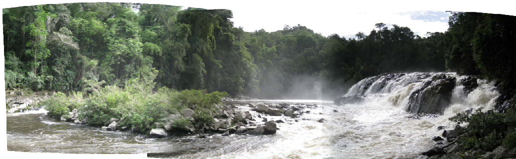
Photo 15.2.1 View of the intake point from 1km downstream
