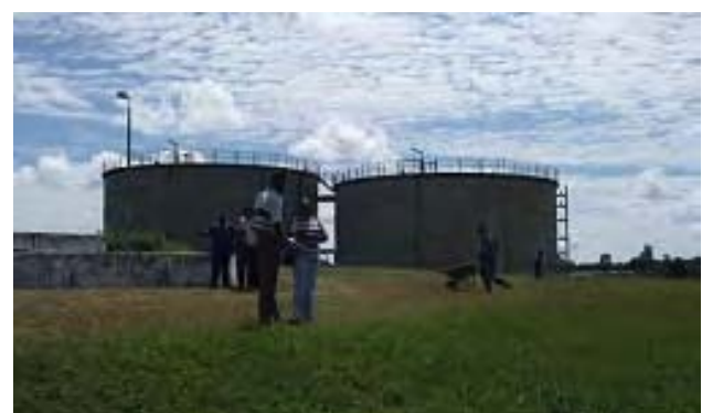
⑪-2 汚泥消化槽
