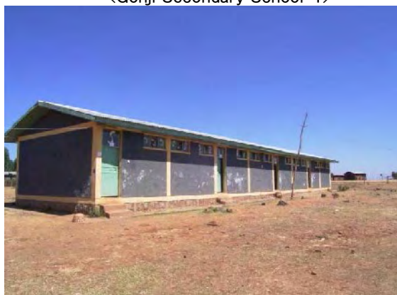
A classroom building of permanent structure
