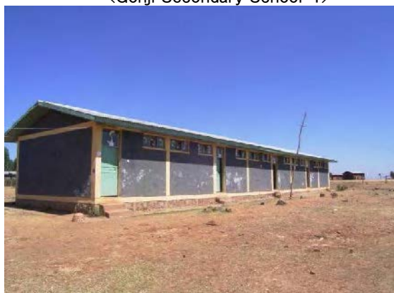
A classroom building of permanent structure
