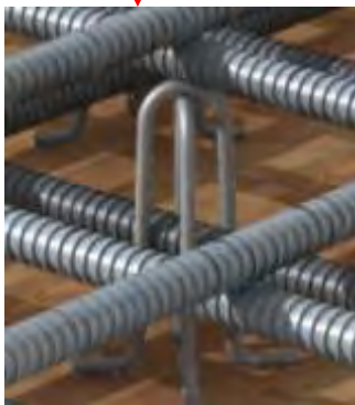
Fig-105 Spacer for upper bar
