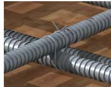
Fig-104 Bar binding
