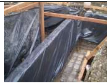
Underground beam: plastic cover to prevent contamination in concrete placing
