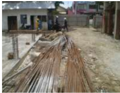
Reinforcing bars left on the ground
