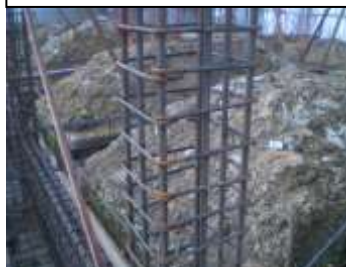
Pillar: neatly assembled reinforcing bars
