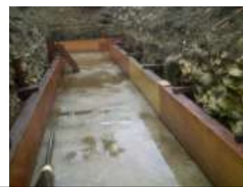
Foundation: formwork with no deformation or gap
