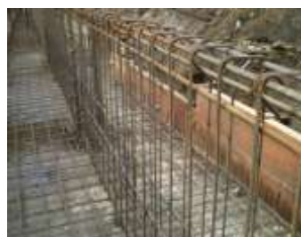
Underground beams: neatly arranged reinforcing bars
