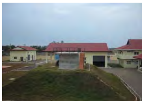
Photo 5: SRWSA Water Purification Plant (Japan Grant Aid Project)
