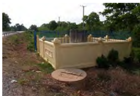
Photo 7: SRWSA Production Well (PW-4) located along Canal
