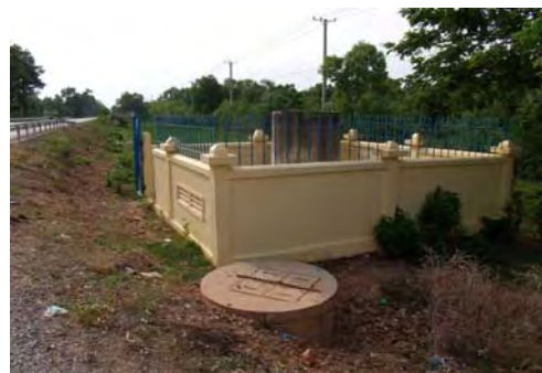
Photo 7: SRWSA Production Well (PW-4) located along Canal
