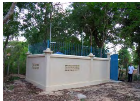
Photo 14: Kravan Monitoring Well (Completion Date: October 2009)
