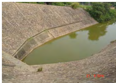
Photo 3: Canal Outlet from West Baray
