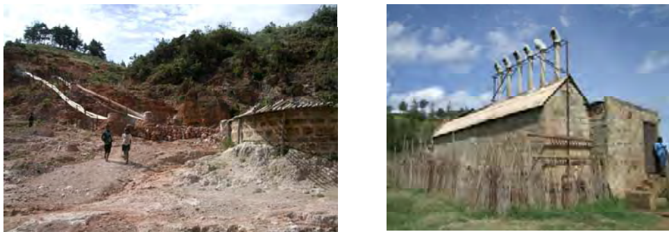
Photo-2.2-2 Direct Use of Geothermal Energy in Eburru area, Kenya (left: Facility condensing water from geothermal steam, right: A Drier house for agriculture products using geothermal hot water)
