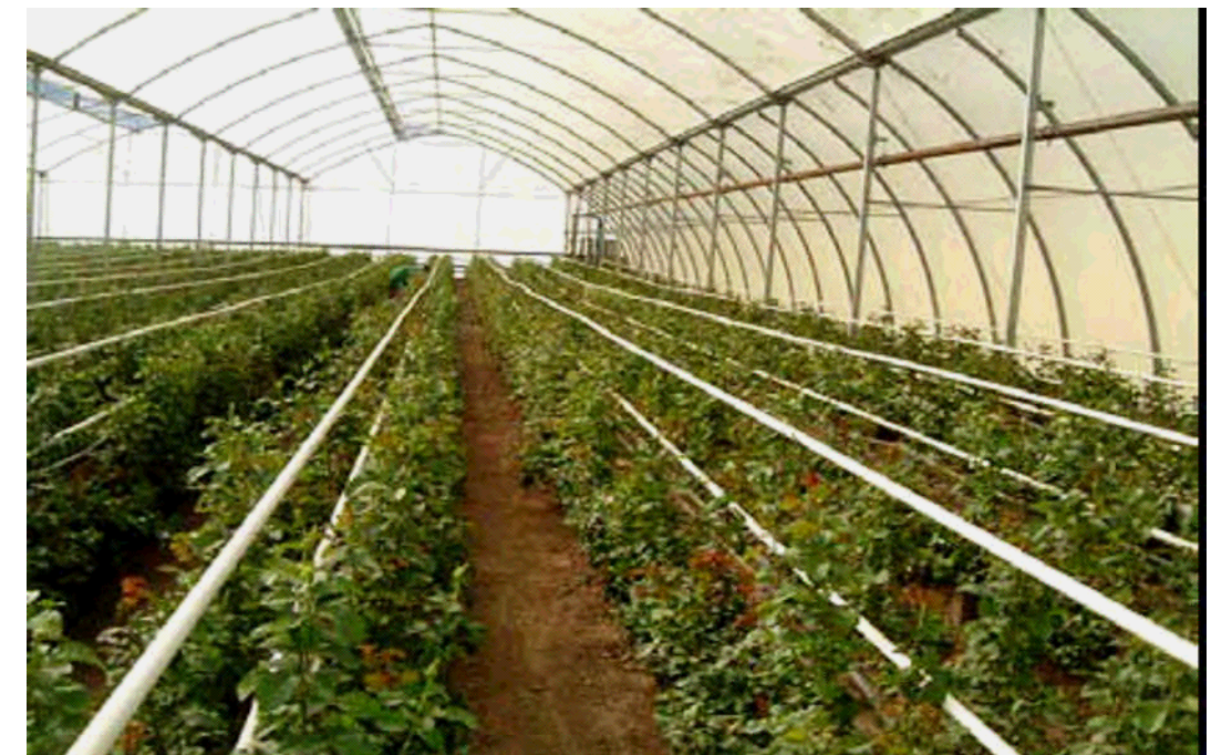
Direct-Use in Oserian Greenhouse utilizing Geothermal Heat
