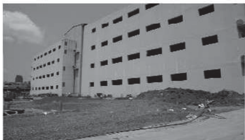
Chong Nonsi WWTP (in operation)
