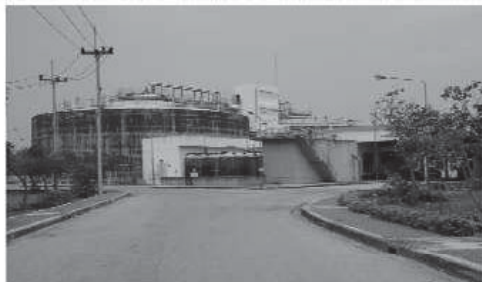
Nong Khaem WWTP (in operation) 2
