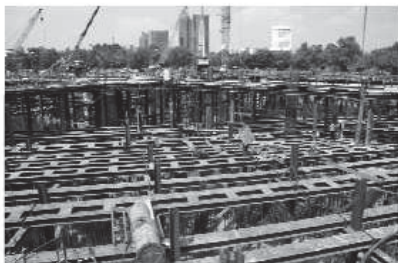
Bang Sue WWTP (under construction)
