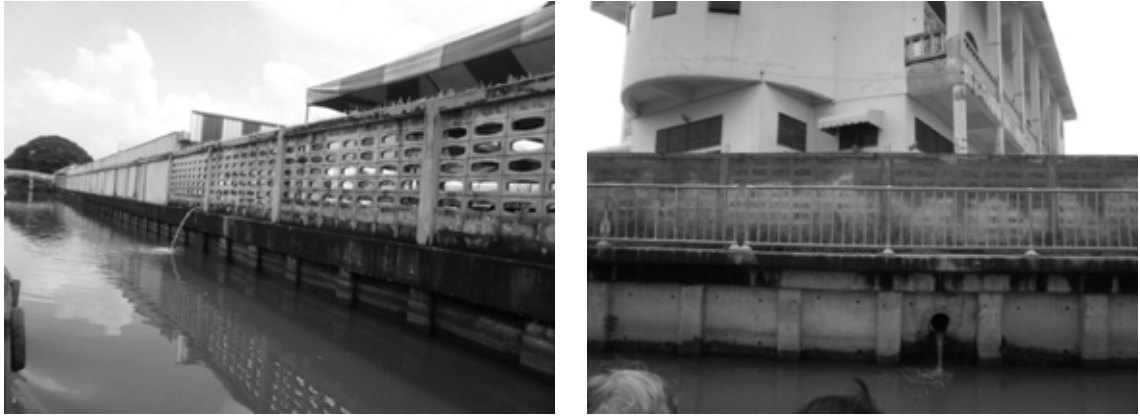
Photo 3.7.2 Direct Discharge of Wastewater from Households to Klong
