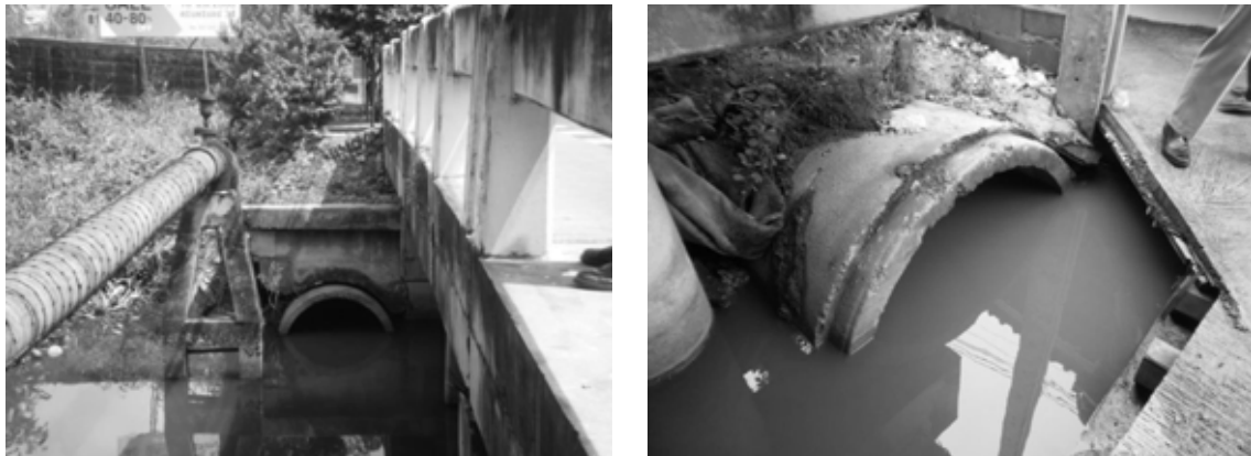
Photo 3.7.1 Submerged Existing Outlets in Nong Bon Treatment Area
