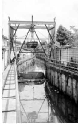
Photo 3.3.1 Vertical Shaft Constructed in Klong
