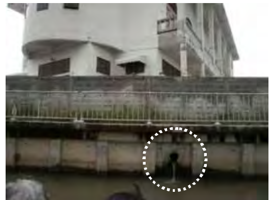
Photo 3.3.2 Direct Discharge from Houses along Klong Khlet
