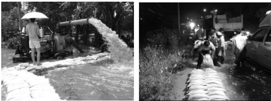
Photo 2.1.2 Emergency Countermeasures (Mobile Pump and Sand Bags)
