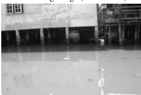
Photo A3.8 Septic Tank
