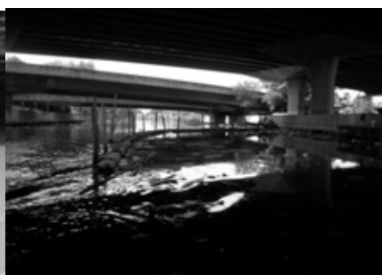
Photo A3.9 Garbage Trap
