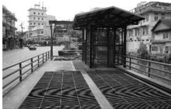
Relay pumping station (pump pit, control panel)
