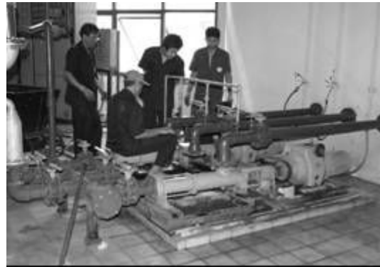
Pump maintenance by BMA staff
