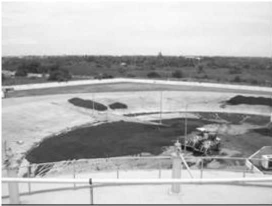
Sludge stock yard
