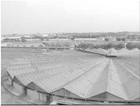
Final sedimentation tank (covered for prevention of algae proliferation)
