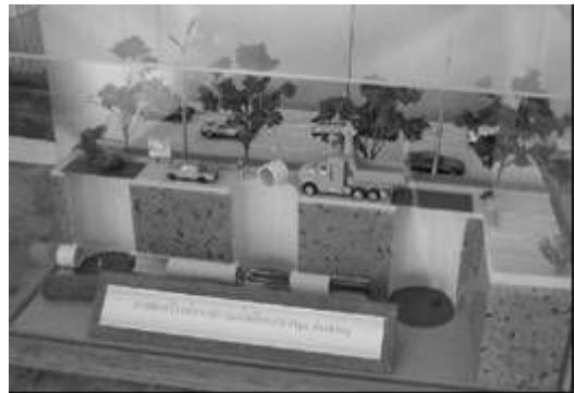
Sewer installation (model)
