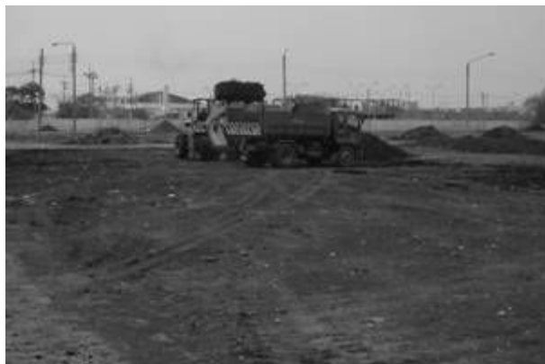
Carrying out of sludge compost
