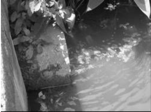
Discharge from interceptor chamber in dry weather
