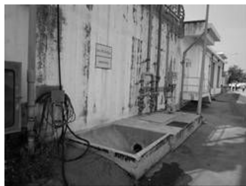
Septic tank sludge receiving pit
