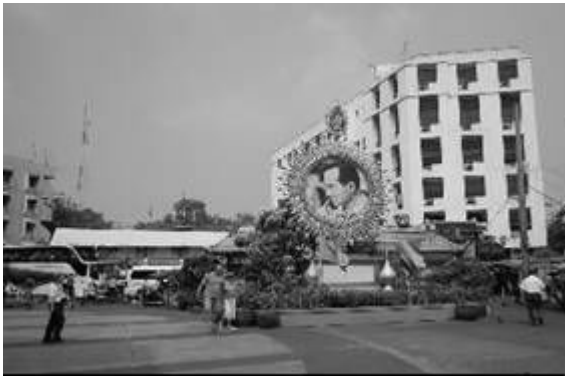
Sipraya WWTP (next to hotel and wharf)
