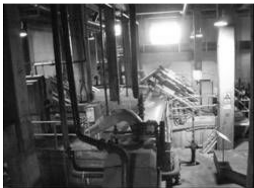
Dynamic separator (swirl grit chamber)
