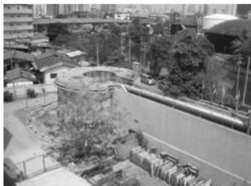
Wastewater pump house
