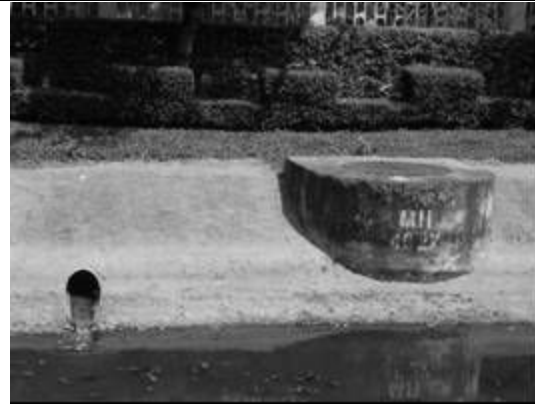
Photo 3.6.2 Untreated Wastewater Discharge near an Interceptor
