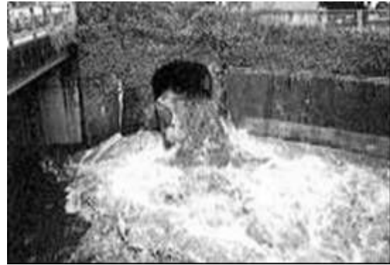
Photos 4.2.1 (left) and 4.2.2 (right) Example of CSO in Japan Dry Weather (Left) and Wet Weather (Right)
