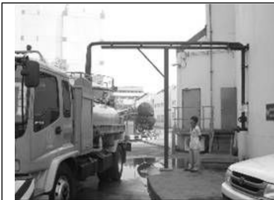
Photo 4.2.9 Use of Treated Wastewater ( Tank Truck)
