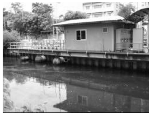
Photo 4.2.8 Existing Storm water Pumping Station (Nara Thiwat Rajanagarindr Street)
