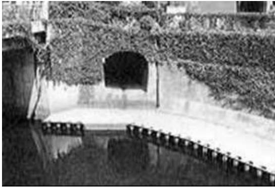
Photos 4.2.1 (left) and 4.2.2 (right) Example of CSO in Japan Dry Weather (Left) and Wet Weather (Right)
