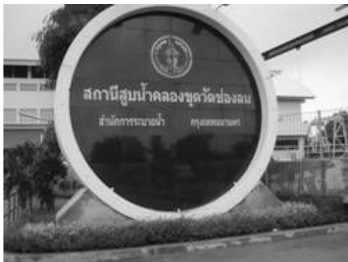
Photo 3.4.7 Entrance to No.7 Makkasan Tunnel Pumping Station
