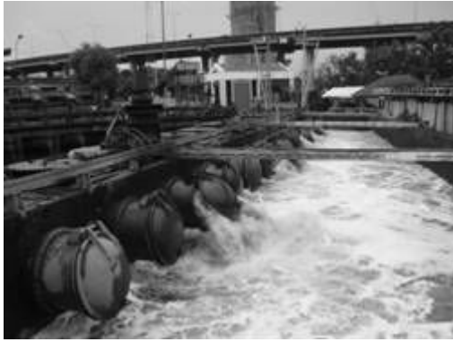
Photo 3.4.1 Phra Khanong Pumping Station
