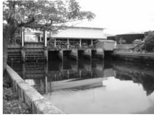
Photo 3.4.2 Chong Nonsi Pumping Station
