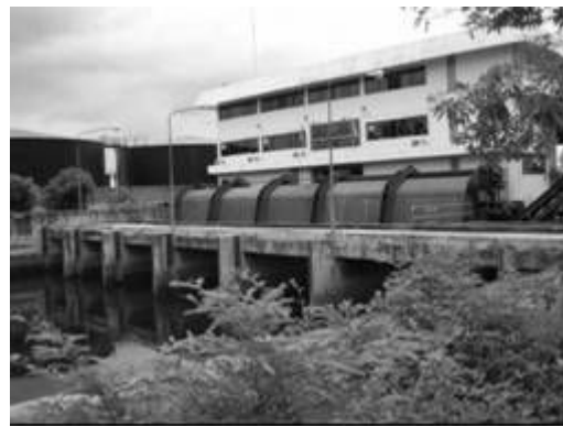
Photo 3.3.2 Dilution of Klong Water System (No.13 Chong Nonsi Pumping Station)
