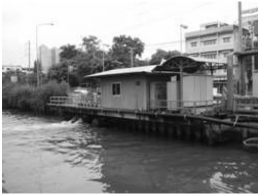
Photo 3.4.3 Existing Storm Water Pumping Station ( along Nara Thiwat Rajanagarindra Street )
