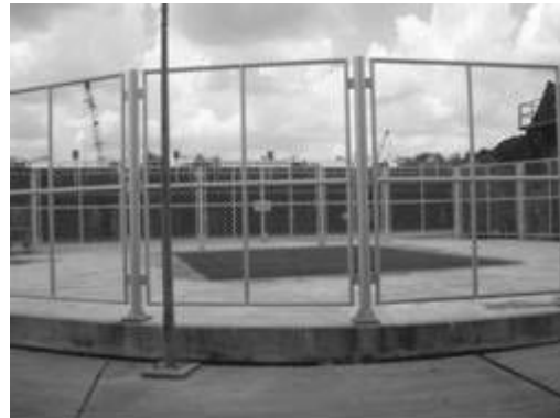
Photo 3.4.6 Manhole at the Beginning of Tunnel, No.6 Klong Saen Saep
