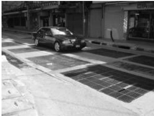
Photo 3.4.5 Manhole Pumping Station at the Beginning of Tunnel, No.1 Sukmvid Soi 26
